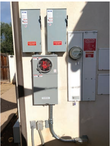
Secondary meter for utility with disconnects.
