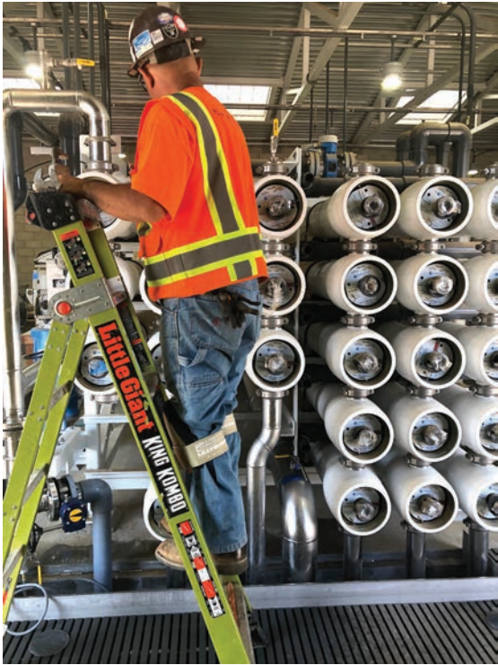
A crewmember works on the reverse osmosis filtration system that will be used to treat the water.
