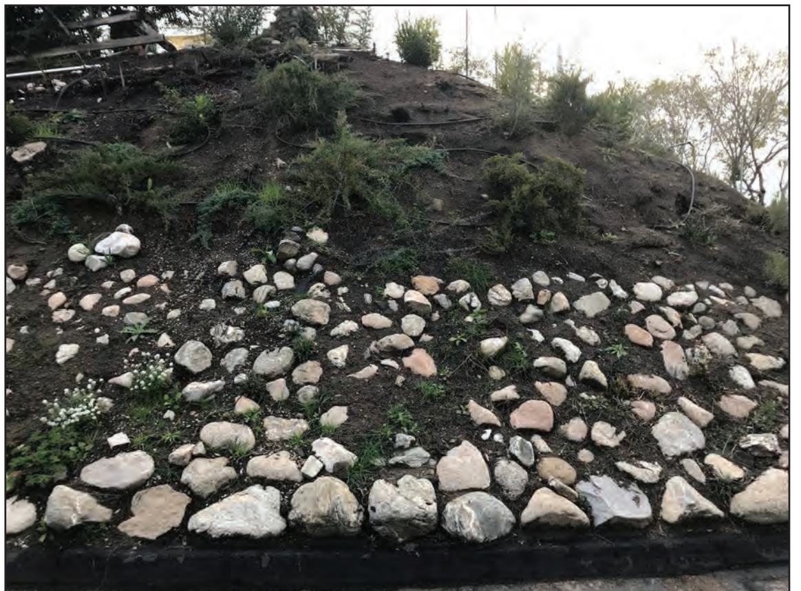
Slope retention can be managed with cobblestones and plantings.
