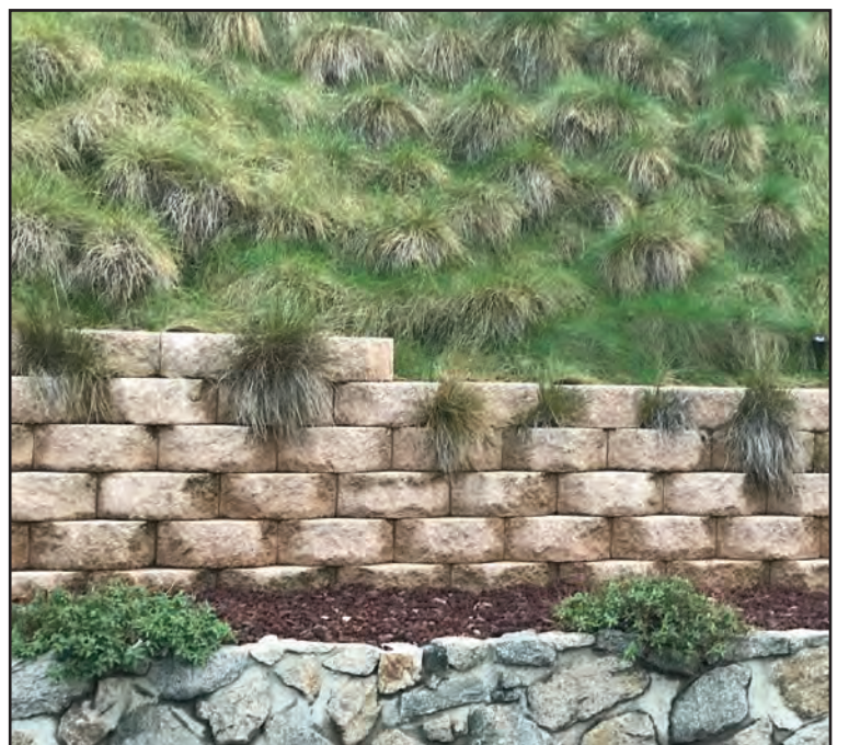
Terraced slope of stacked blocks and plantings keep a hillside from eroding.
