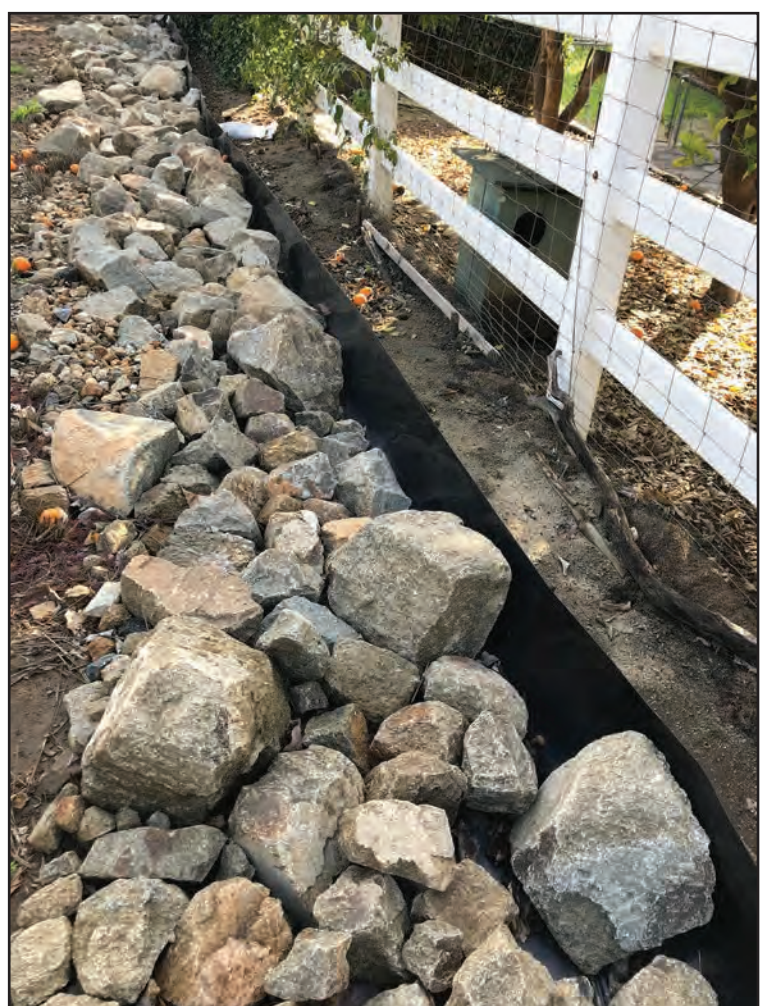
Assorted sizes of boulders and rip rap that channel runoff rainwater can aid in erosion control.
