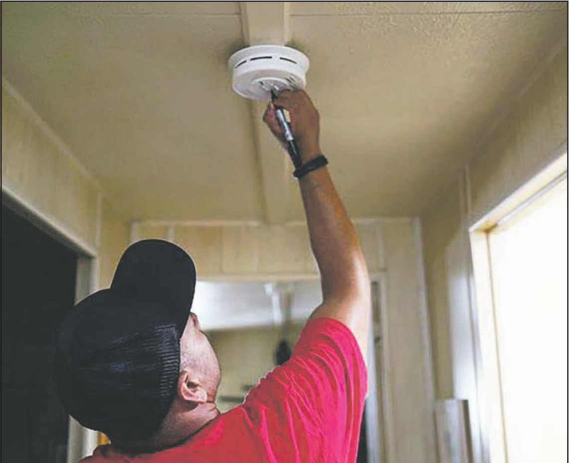
A man tests a newly installed smoke alarm.
