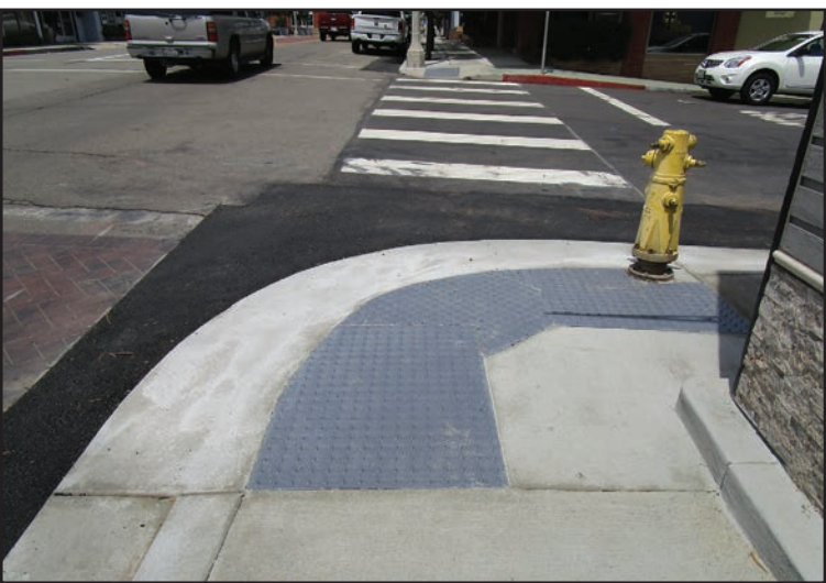
The county put in a handicapped accessible curb ramps on each side of Hawthorne Street at Main Avenue besides removing the tree that blocked sight of traffic on the southeast corner.
