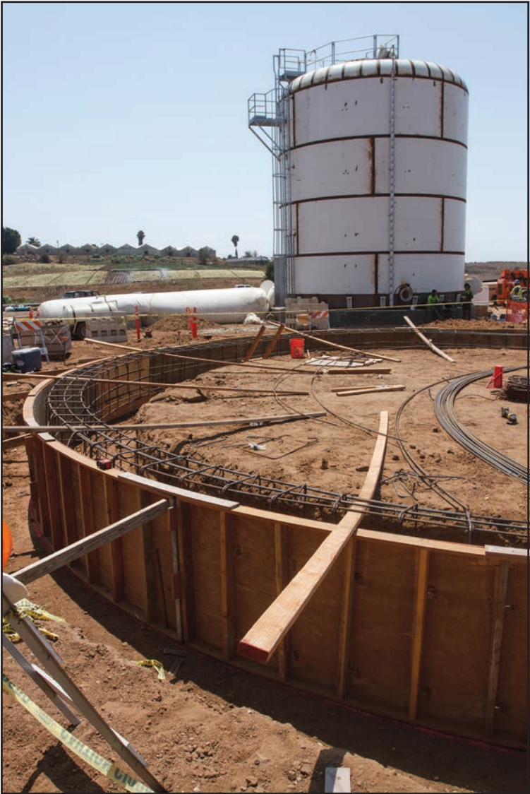
The foundation of another water storage tank is constructed at the new FPUD water treatment plant.
