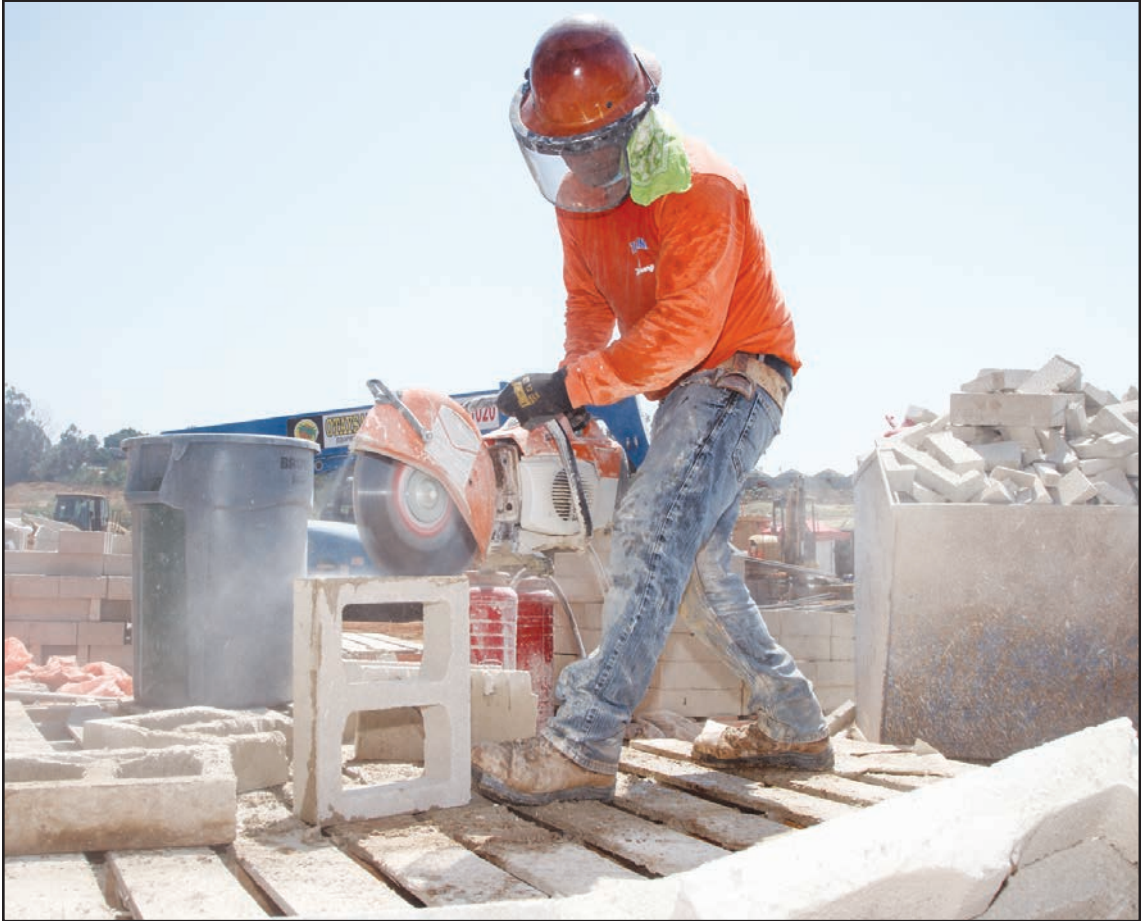
A construction worker cuts cement blocks to size for the new FPUD water treatment plant in Fallbrook.
