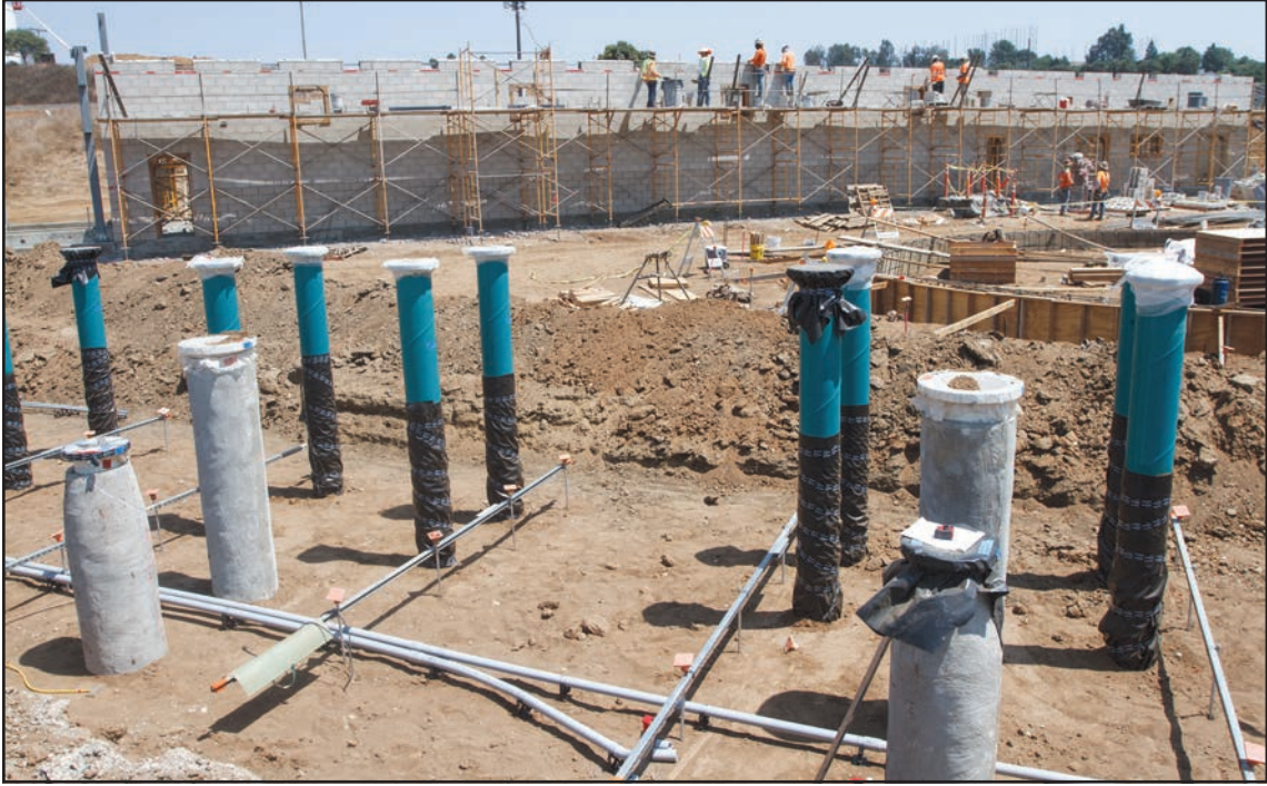
Piping for processing the water and a building where reverse osmosis will take place at the FPUD water treatment plant are under construction at the end of August.
