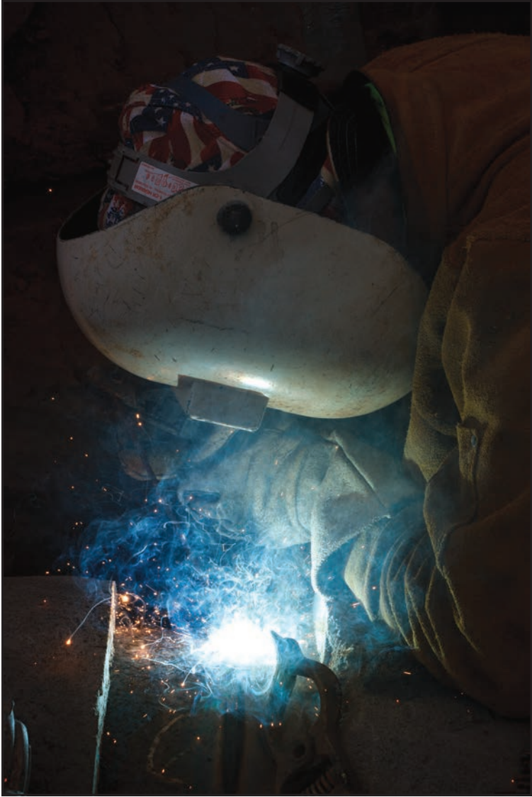
A welder seals two sections of water main pipe along Palomino Road as part of the Santa Margarita Conjunctive Use Project.
