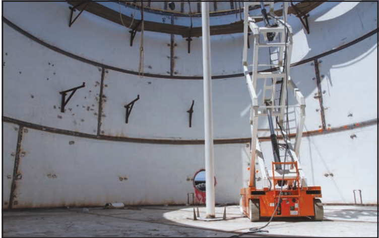
Construction crews work to complete the roof of a water tank at the new FPUD water treatment plant project in Fallbrook.
