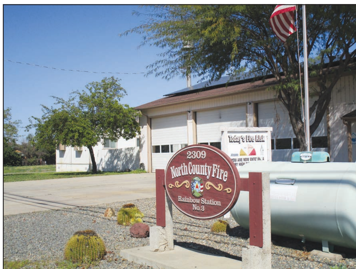
The fire station in Rainbow is getting a new modular building with about 2,000 square feet of living space as the former all-volunteer station did not have living quarters.
