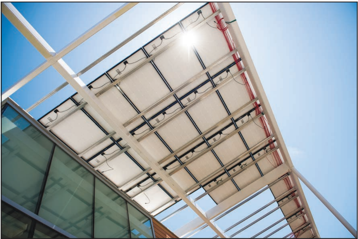
A 180-kilowatt photovoltaic array was installed this summer on the new maintenance and operations building at Palomar College, which has won numerous awards for its energy-saving design features.
