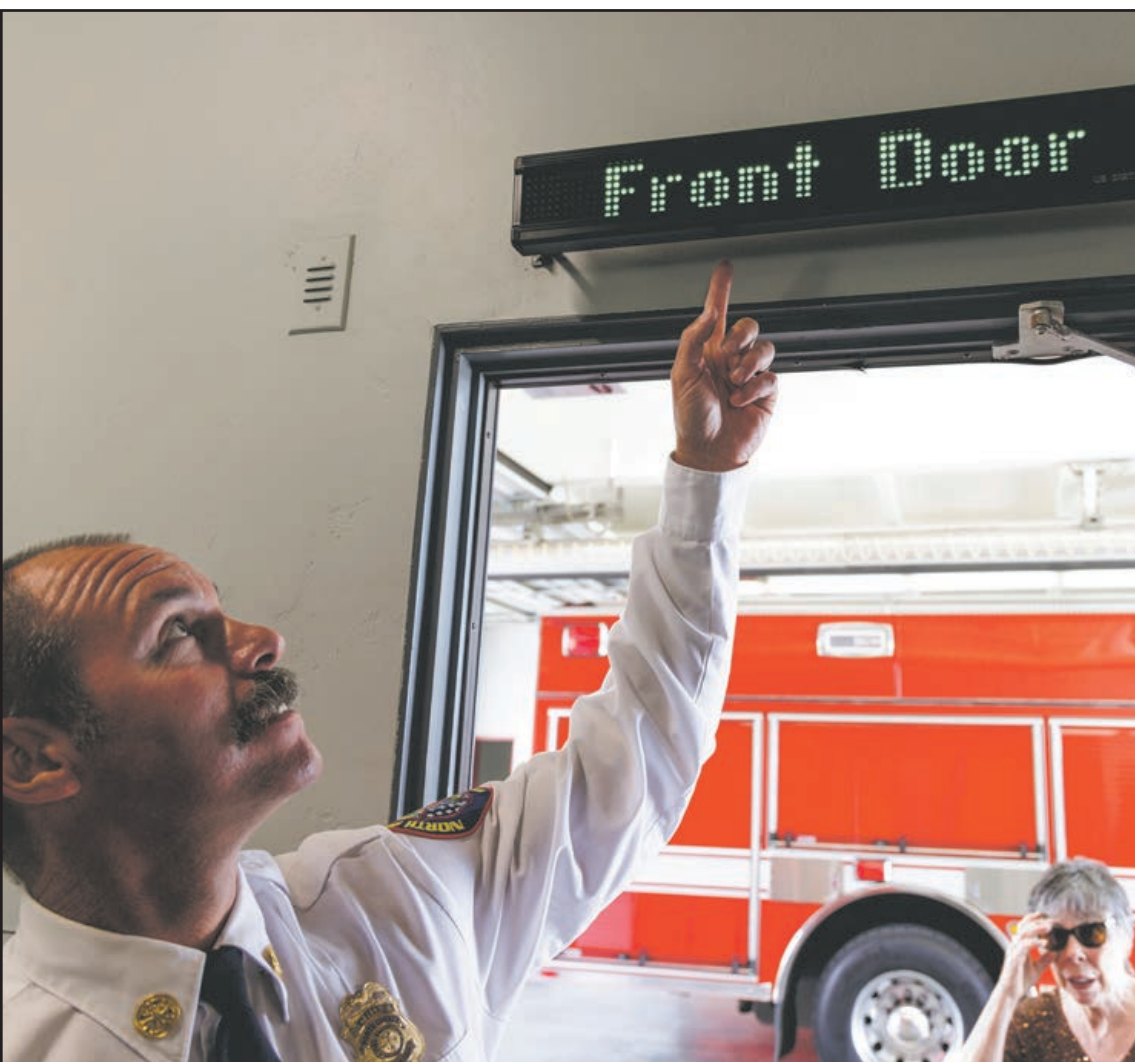
NCFPD Chief Keith McReynolds points out Fire Station 2's new LED alerting system during a tour of the facility.
