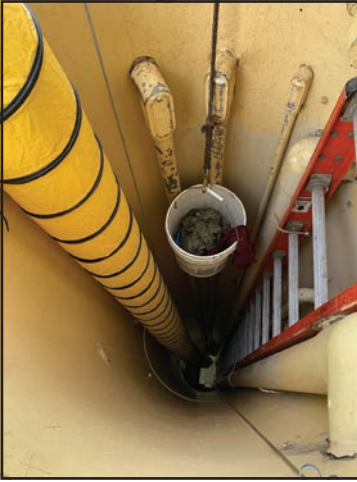
A bucket. Village News/Rainbow Water photo of 'flushable' wipes is being pulled up from a lift station after they got stuck in the sewer system.
