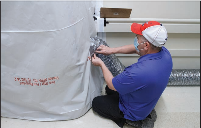
Temecula Valley Hospital HVAC technician Jason Sovacool adjusts the negative air flow vent to contain airflow from a restricted area where suspected COVID-19 patients are treated safely.
