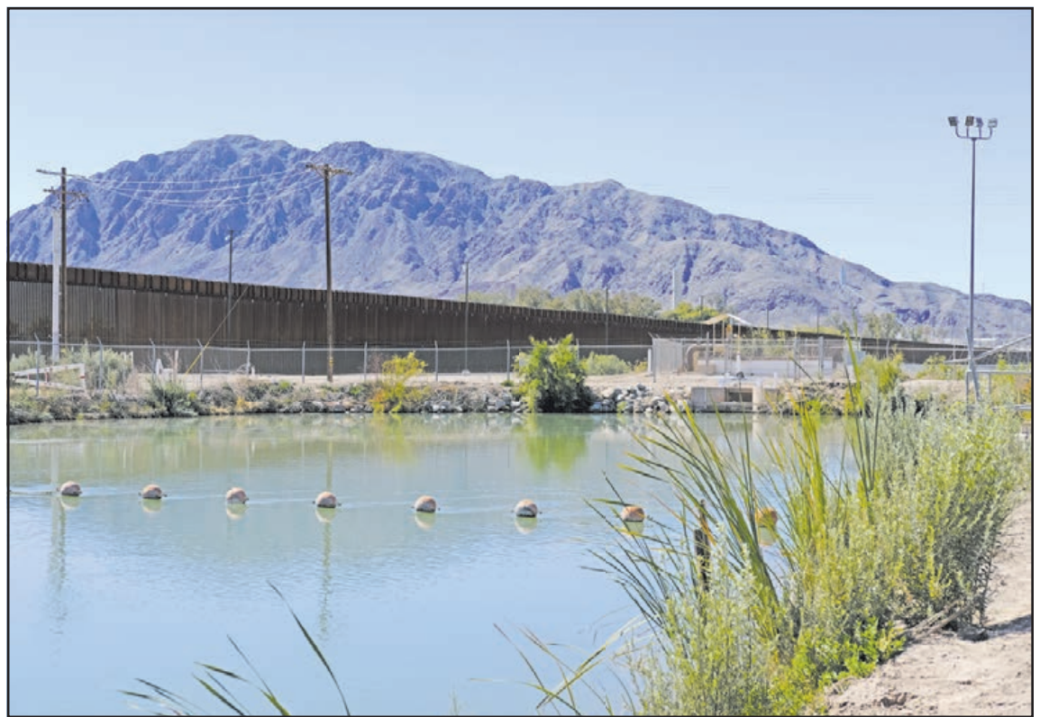
The All-American Canal runs along the U.S.-Mexico border and delivers water from the Colorado River to the Imperial Valley. Farmers in the valley use most of California's entitlement to the river. Village News/Caleb Hampton photo
