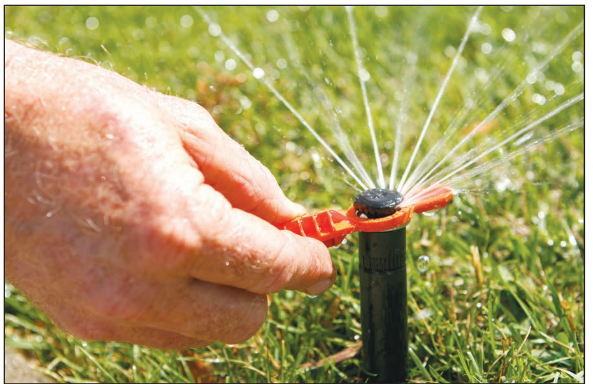
Bob Butler of Butler Landscape demonstrates how to adjust a Hunter MP Rotator sprinkler at a home in Bonsall.
