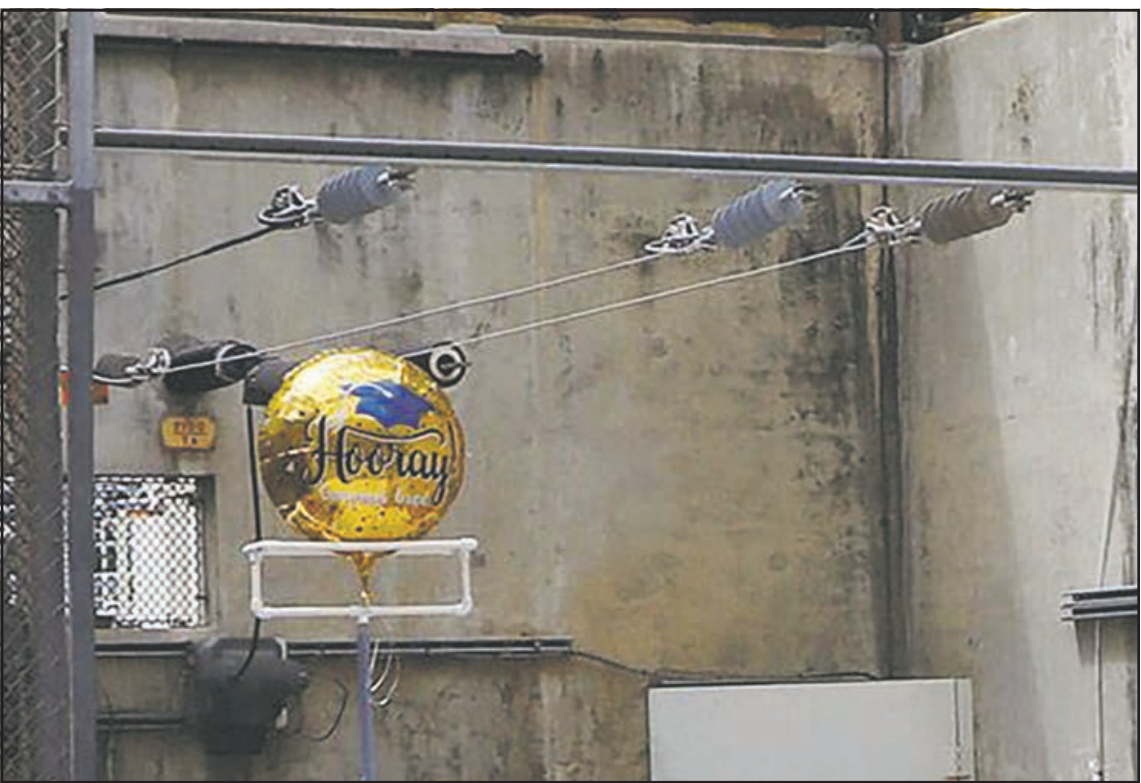
Regular mylar balloons can cause power outages and fires when they get tangled up in power lines because the foil conducts electricity. Village News/Courtesy photo
