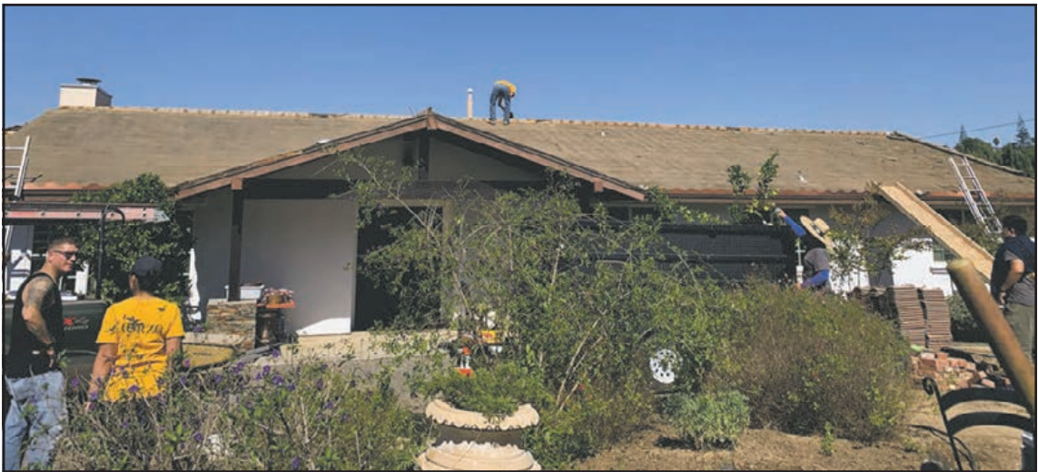
A volunteer on the roof helps take ridge tiles off the roof after all the other tiles have been removed.
