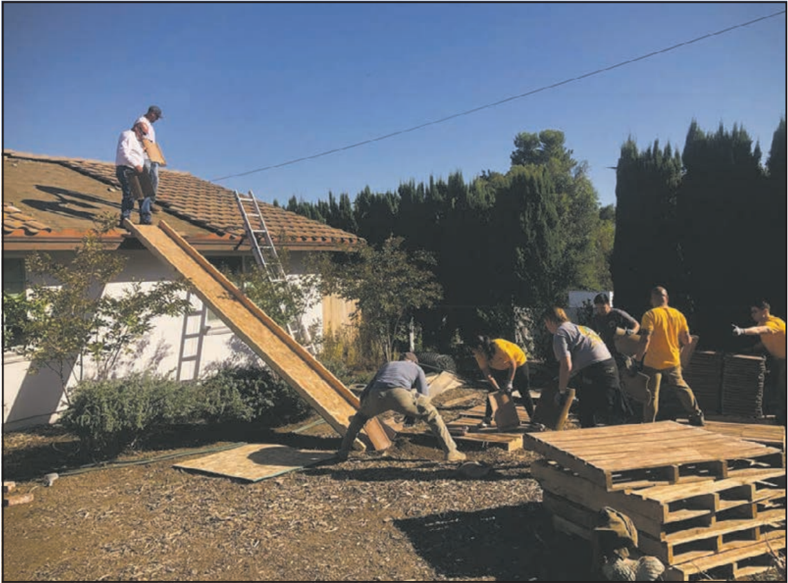
A slide is used to transport the heavy concrete tiles from on top of the roof to the people on the ground who were stacking them. The volunteers created a bucket brigade type line to help carry the heavy tiles from the top of the roof to the pallets on the ground.
