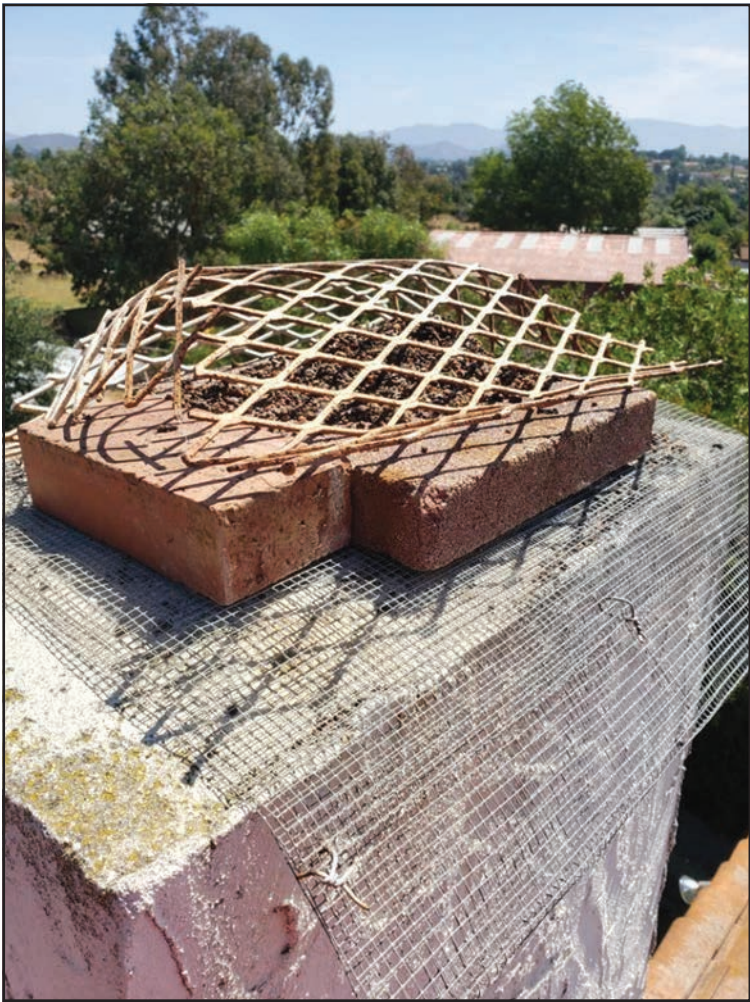
This McGyver-style spark arrestor works but is not up to code.
