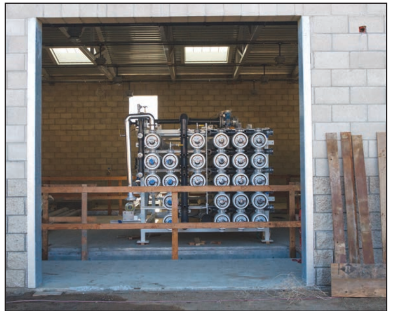
A series of reverse osmosis water treatment filters is seen during a tour of the new FPUD water treatment plant construction.
