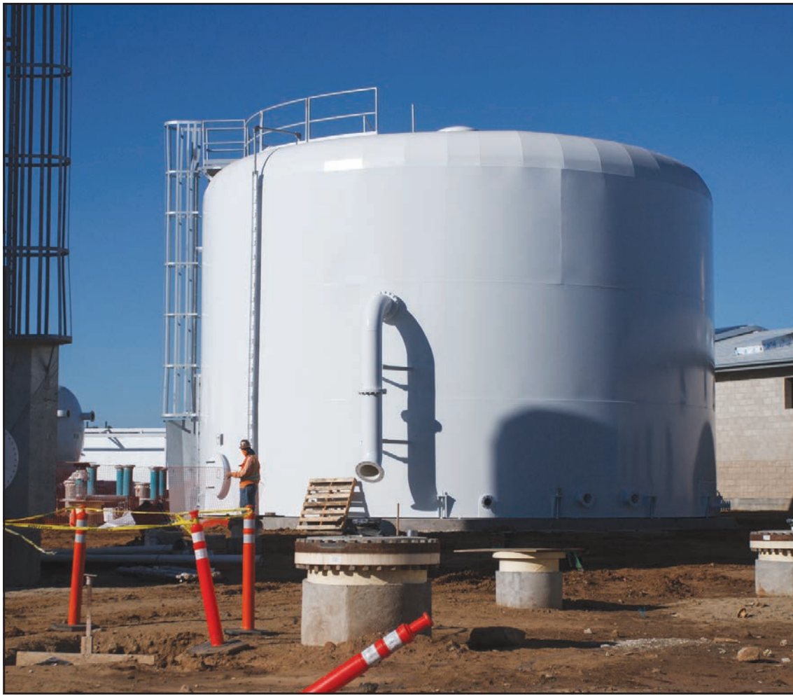
New water tanks of different sizes are installed at the FPUD water treatment plant construction site.
