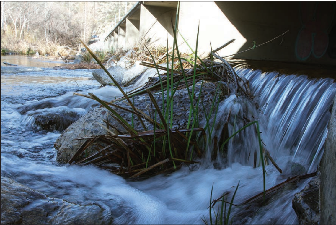
The Sandia Creek Drive bridge currently blocks fish passage to 12 miles of upstream habitat. As a result, adult steelhead cannot reach their natal spawning grounds in the river’s headwaters.
