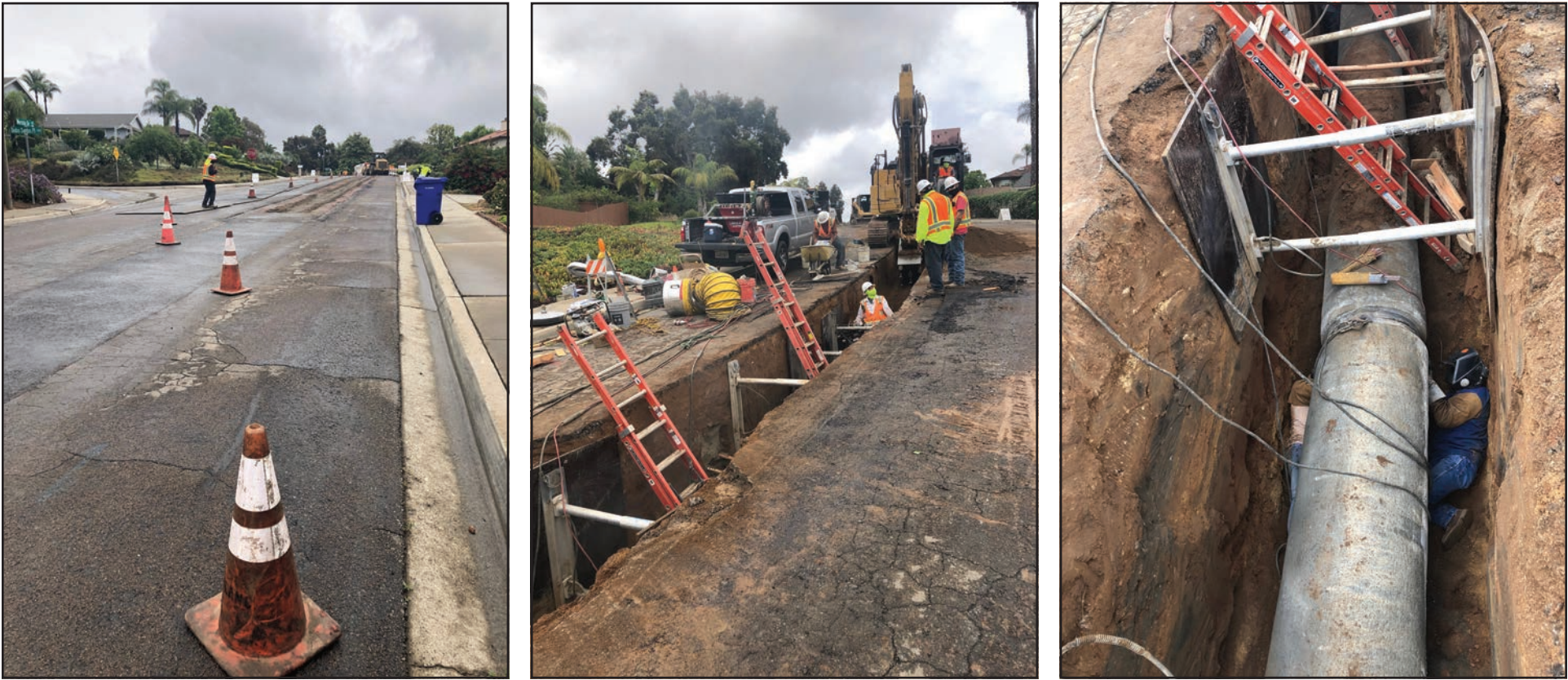
Construction of the first section of pipeline on Merida Drive is for the Santa Margarita River Conjunctive Use Project. This segment of pipeline between Alturas and Mission roads is about 4,500 linear feet and is 35% installed. The project is expected to be delivering water to Fallbrook taps in early 2022.
