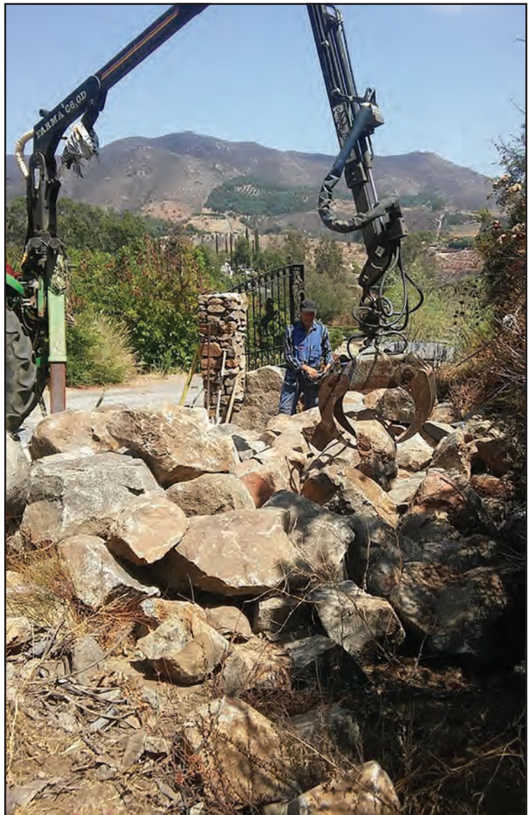
StenErik Rolfo uses the remote control crane he invented to move the heavier stones for wall building.
