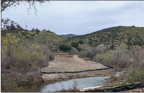
Downstream of the existing box culvert crossing is the fully cleared path for the new 574 ft steel bridge, looking from the north (left) and south (right) sides of the river channel.
