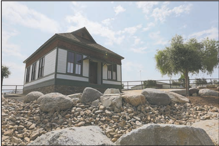
Looking east, this shot shows the new bioswales that capture rain and run off.
