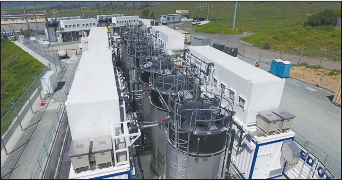
The vanadium redox flow battery based at a San Diego Gas & Electric substation is again breaking new ground as it is being tested as a means to help achieve zero-emission microgrids.
