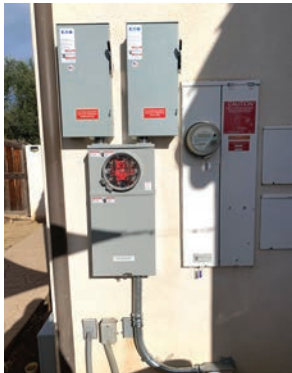
Secondary meter for utility with disconnects.
