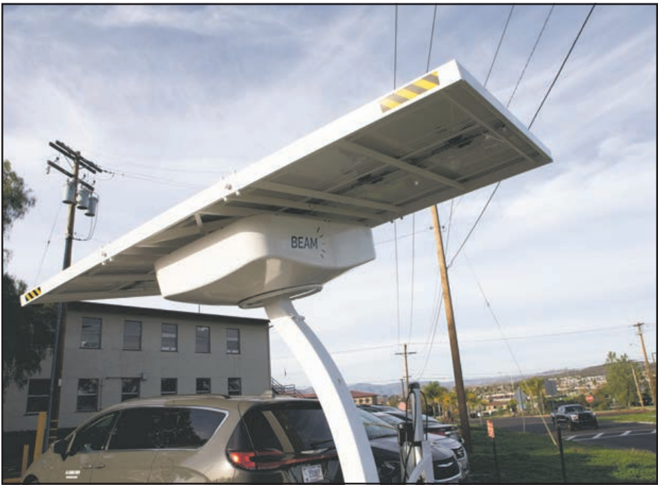
A Beam electric vehicle charger operated by Marine Corps Installations West's South West Region Fleet Transportation office sits in a parking lot in the 14 Area of Marine Corps Base Camp Pendleton, Jan. 12. The SWRFT office recently acquired the solar-powered charging stations to test with their fleet of government vehicles on several installations in the region. U.S. Marine Corps photo by Lance Cpl. Shaina Jupiter
