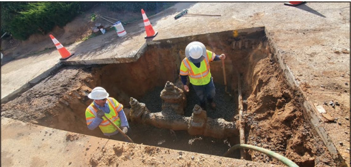
Fallbrook Public Utility District crews are working to replace an old underground water feed that failed Friday night. They are replacing a junction where a 12-inch water pipe and 2 8 inch water pipes come together under the street.
