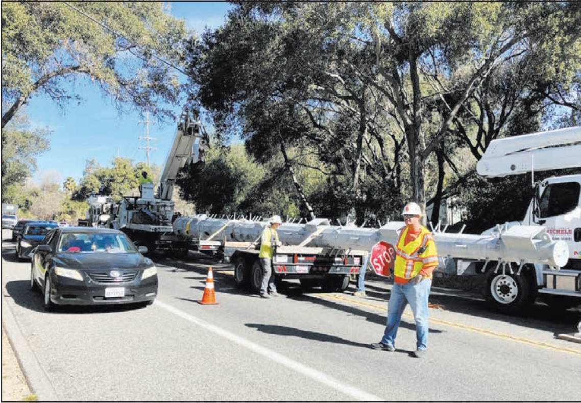
Workers prepare to lift a steel power pole that was subsequently installed along South Mission Road. Village News / Tim O’Leary photos
