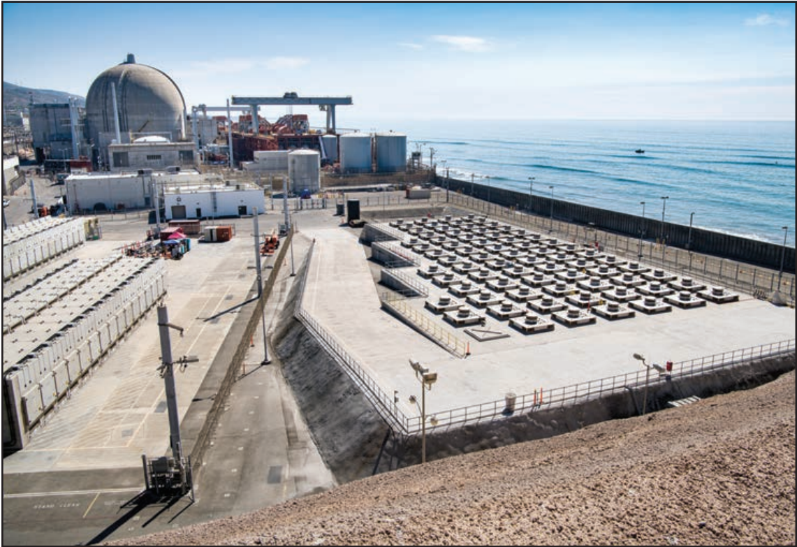
At San Onofre Nuclear Generating Station, the Orano TM System, left, holds 50 spent fuel canisters while the Holtec System, right, holds 73 spent fuel canisters. The decommissioning Project is halfway done.
