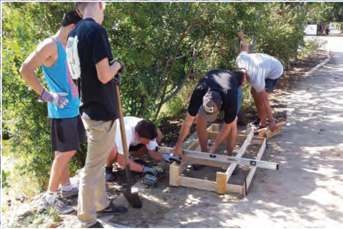
Members of the Riverview Church Youth Group build forms to pour cement into while making foundations for new benches.
