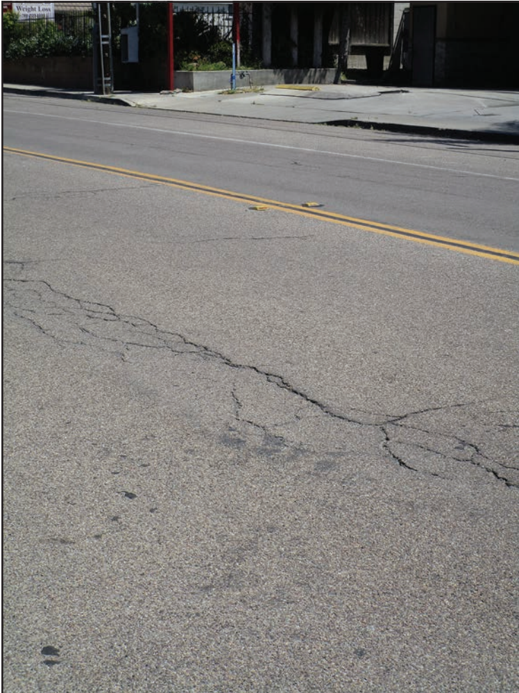
This portion of East Alvarado Street is one that will be getting an asphalt concrete pavement overlays to repair extensive cracking.
