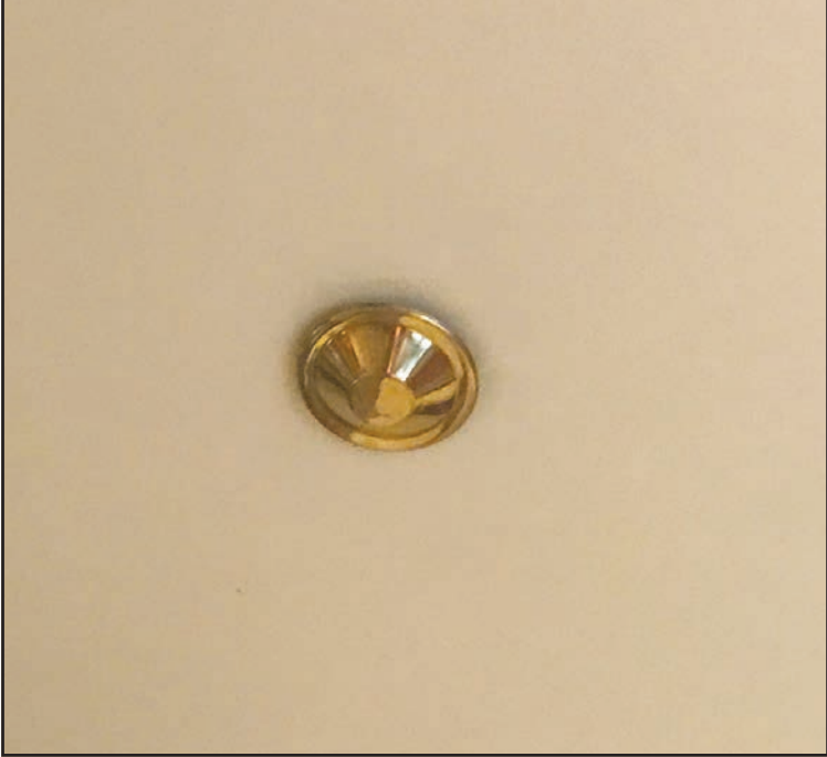
An interior sprinkler system in the ceiling can help put a home fire out.
